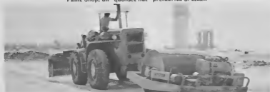
The Hyster compactor pulled by Caterpillar prepares new road area. The engine at the rear of the unit moves roller sideways as it is pulled, to smooth and pack surface.
